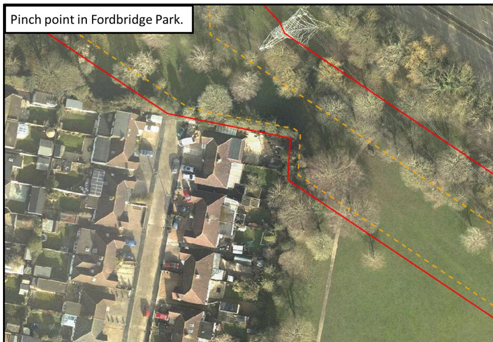
Illustration 3.1: Pinch point in Fordbridge Park
